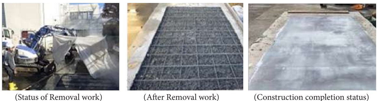
Figure 2. Removal work by Water Jet method
